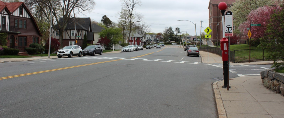
Figure 4B: Church St and Centre St opposite South St looking towards the Centre/West Rox Pkwy rotary
