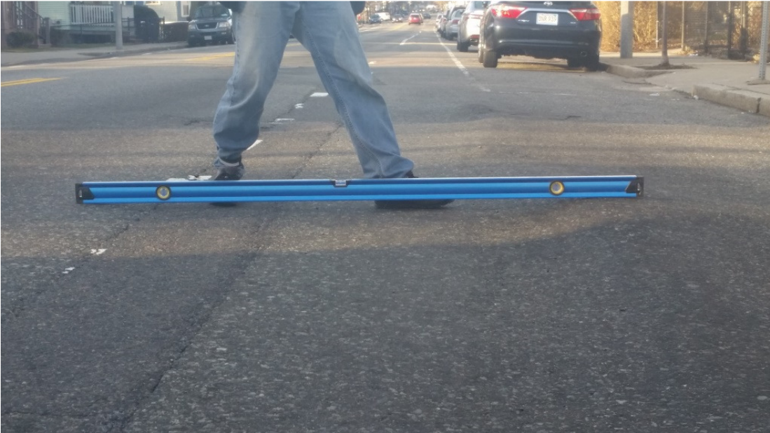
Washington St. Southbound, north of Granfield Ave. March 2016
